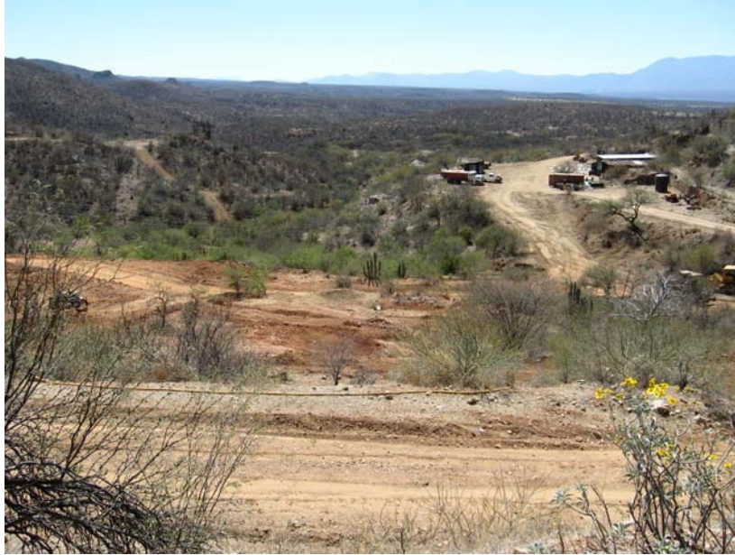
Photo 5: View from the mine portal to the rest of the project. Prior Mill Facility (now used for Core Storage)
